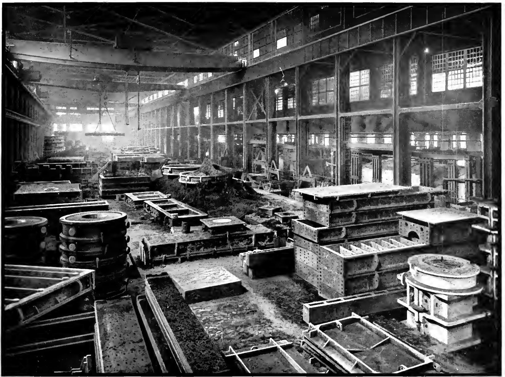
View in Steel Foundry
